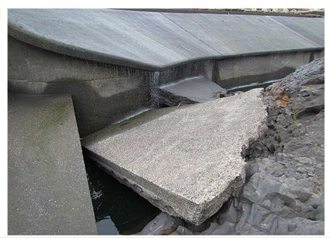
• <u>091820 willamette falls fishway 5 odfw</u> - The failed apron has been demolished and the site is prepped for placing a new concrete slab.
