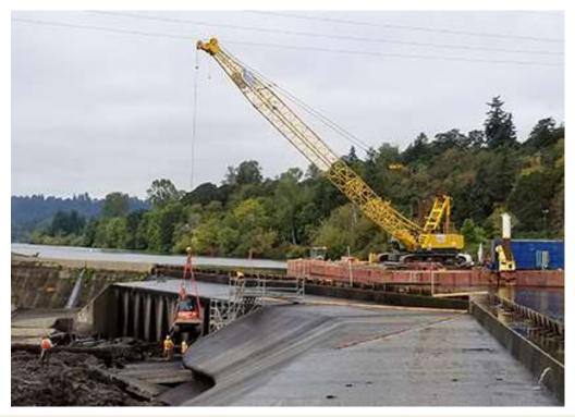
• <u>091820 willamette falls fishway 4 odfw</u> - The barge crane lowers a mini excavator to the site to begin demolition of the failed slabs at Leg 2.
