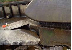
091820 willamette falls fishway 2 odfw - The spill apron at the base of the fishway is dislodged and the gravel under the slabs has scoured away. Without this protection in place, the fishway is at risk for damage.
