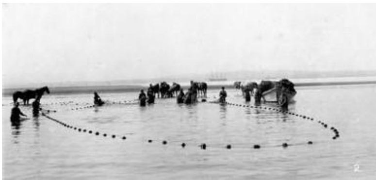
Seine nets hang vertically in the water, with weights at the bottom and floats keeping them upright. Columbia River Maritime Museum
